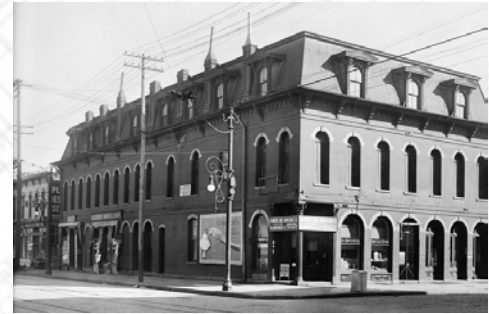
1916 | Constitution Hall at 15th and Blake Streets, where Colorado's constitution was drafted by delegates in 1875. 1521-1523 15th Street is visible at the far left with "SEEDS" sign which was found in the attic, restored, and now hangs in the residential loft.
