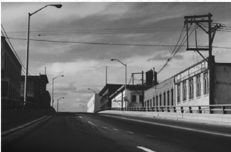
1985 | View of the 15th Street viaduct from Blake Street. The ramped structure rose two stories over the Platte Valley railyard and was demolished in 1991. 1521-1523 15th Street is at far right with its third facade, altered some time in the late 1930s.
