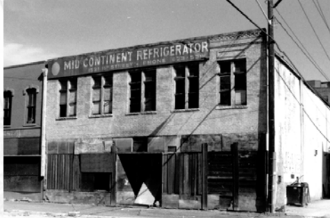
1991 | Photo taken after the 15th Street viaduct was demolished to make way for the 15th Street Pedestrian Mall. The paint on the brick was removed, and the storefront was rebuilt. The metal parapet sign was removed and re-installed downstairs.
